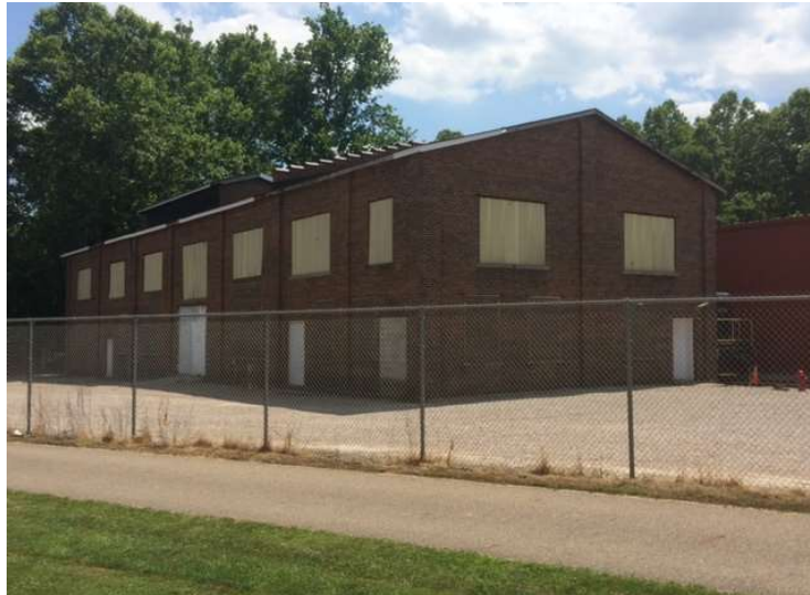
Nelsonville, 2016. Salvaged HVRR machine shop building, waiting to be repurposed. The roundhouse sat at the far end to the east. Photo taken by author from the north side, on the former site of Nelsonville Yard.
