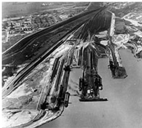
C&O Coal Docks and adjacent terminal yard at Toledo.
