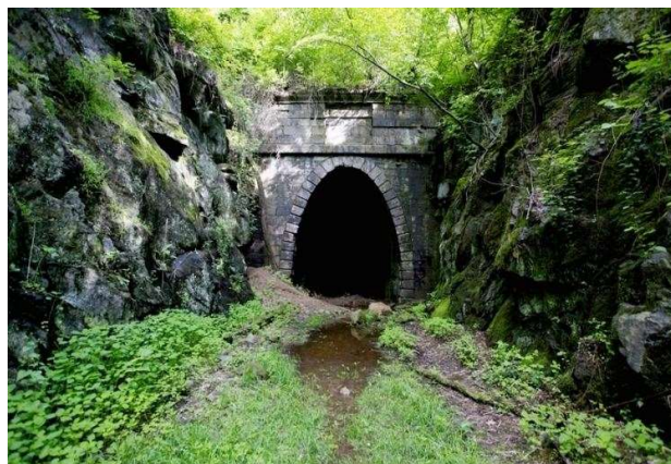
The west portal of the 4,200-ft. C&O Blue Ridge Tunnel, at Rockfish Gap near Crozet, Virginia, completed in 1852. This tunnel, now on a hiking trail, was replaced in the 1940s by a larger bore nearby with a lower grade.
